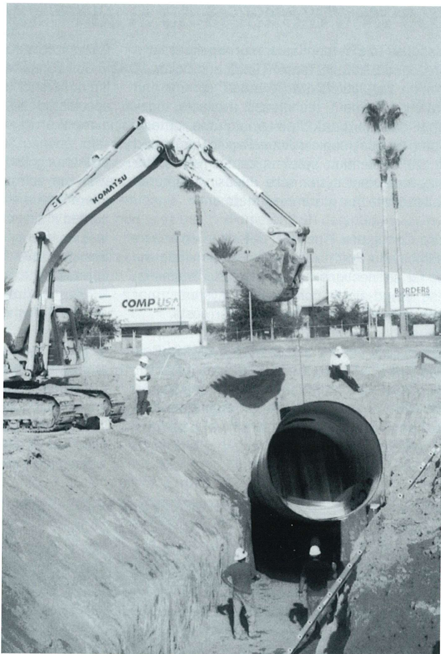
Four feet of cover is required in areas where pipe is subject to construction loading.
