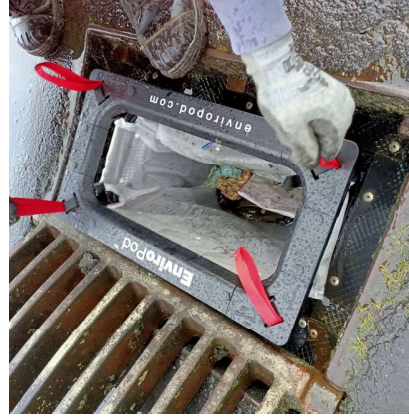
Figure 4: LitttaTrap seen with 1mm liner installed to target micro-plastics such as plastic pellets. Hand maintenance shown.
