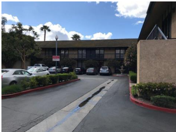
5. View of the typical structural view of the subject property
