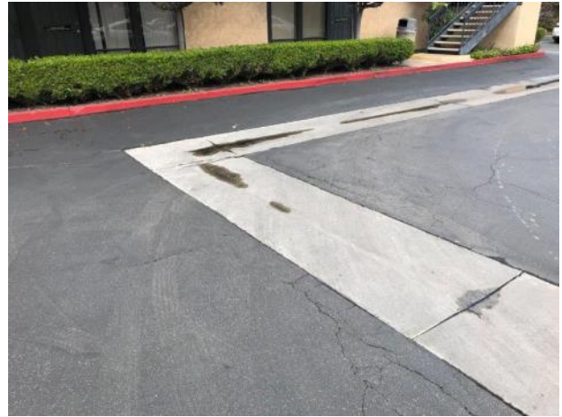
20. View of the concrete swale for water drainage in the parking lot
