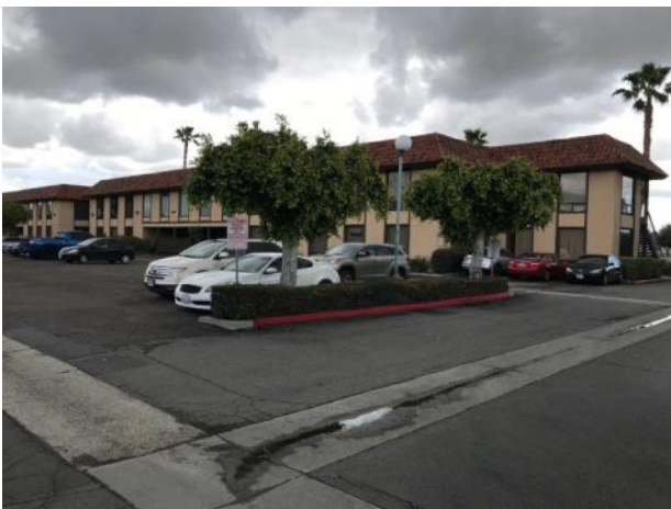
21. View of the eastern adjacent multi-tenant commercial office structure
