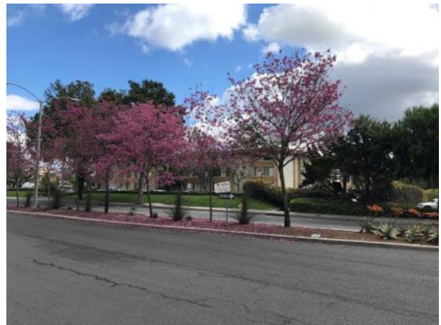
24. View of the northern adjacent multi-family housing structure
