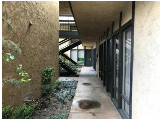
18. View of the first floor walkway and stairway to the second level
