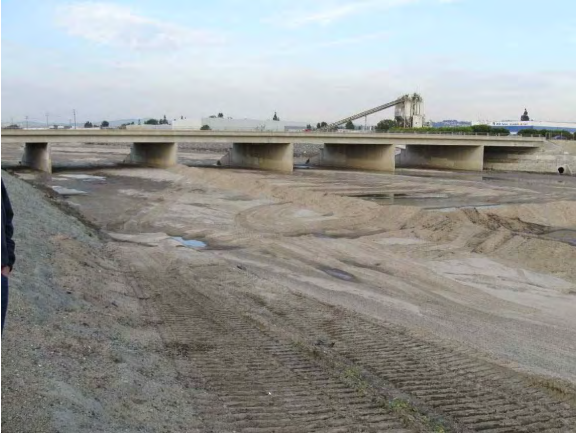
Figure 14-2: Santa Ana River, looking upstream in the vicinity of Ball Road. Here the river, with side levees and a soft bottom, is typically dry during non-storm conditions.
