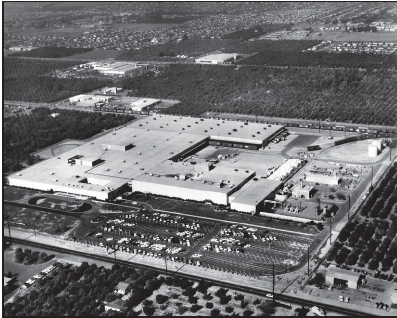
Image 5. Aerial view of the Kimberly-Clark plant, view toward the northwest, showing original configuration of the building and landscape, undated. Source: Albert Launer Memorial History Room, Fullerton Public Library.
