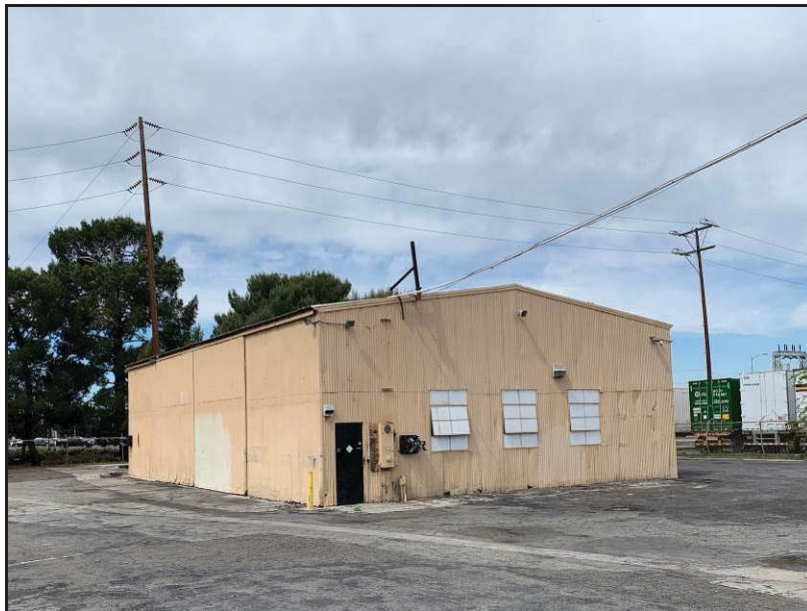
Image 6. The south and east façades of the warehouse, view toward the northwest.
