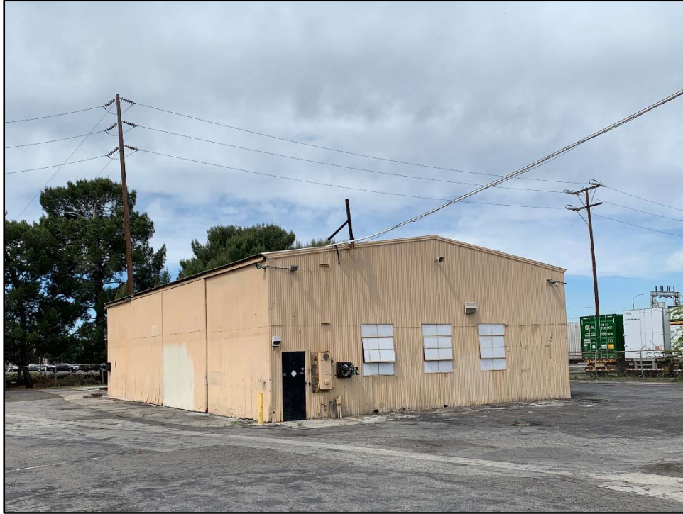
Figure 45. The south and east façades of the warehouse, view toward the northwest.
