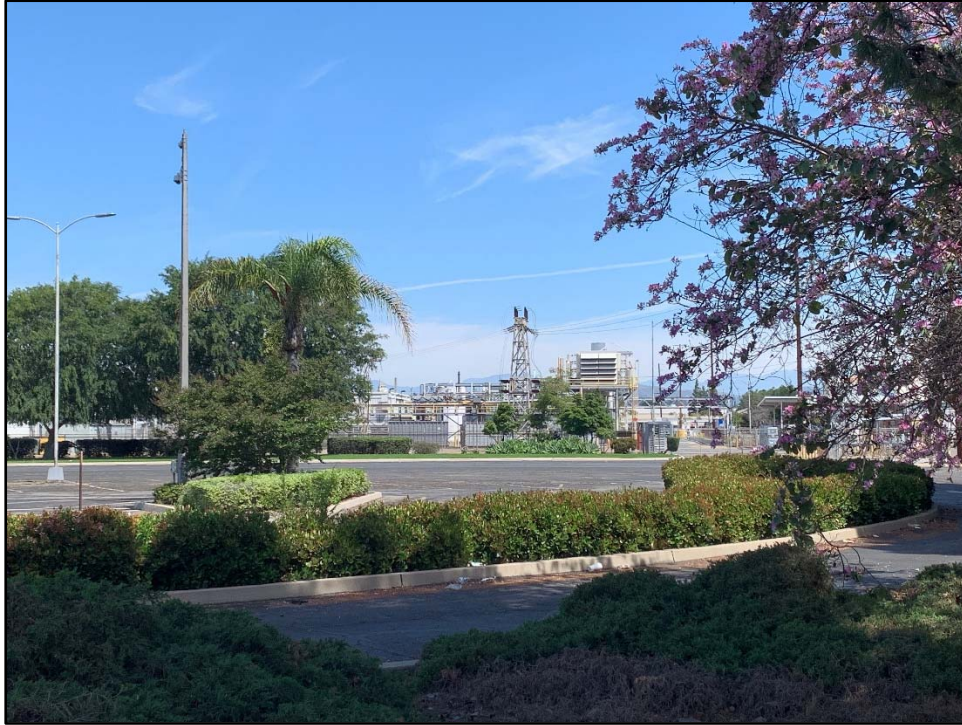
Figure 26. Distant view of the industrial structures to the east of the main building, view toward the north.
