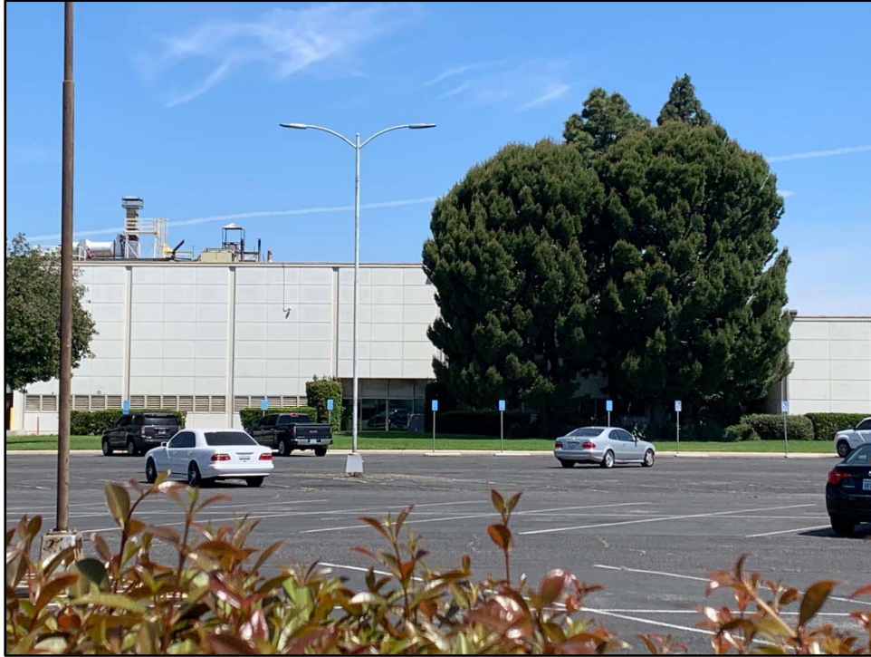
Figure 24. The east end of the south façade, view toward the north.
