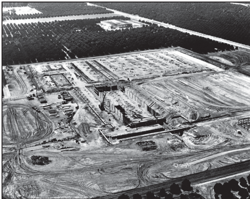
Image 2. The Kimberly-Clark Fullerton Mill under construction, 1955.
