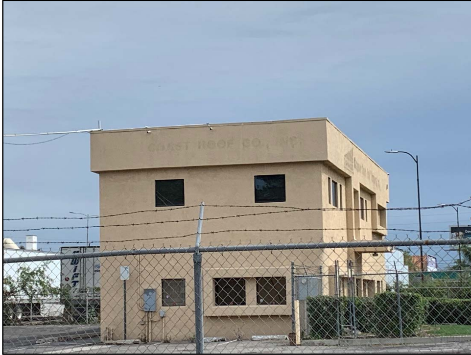
Figure 43. The west façade of the office building, view toward the east.
