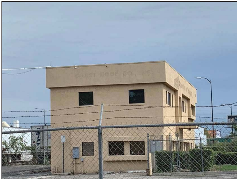
Image 4. The west façade of the office building, view toward the east.
