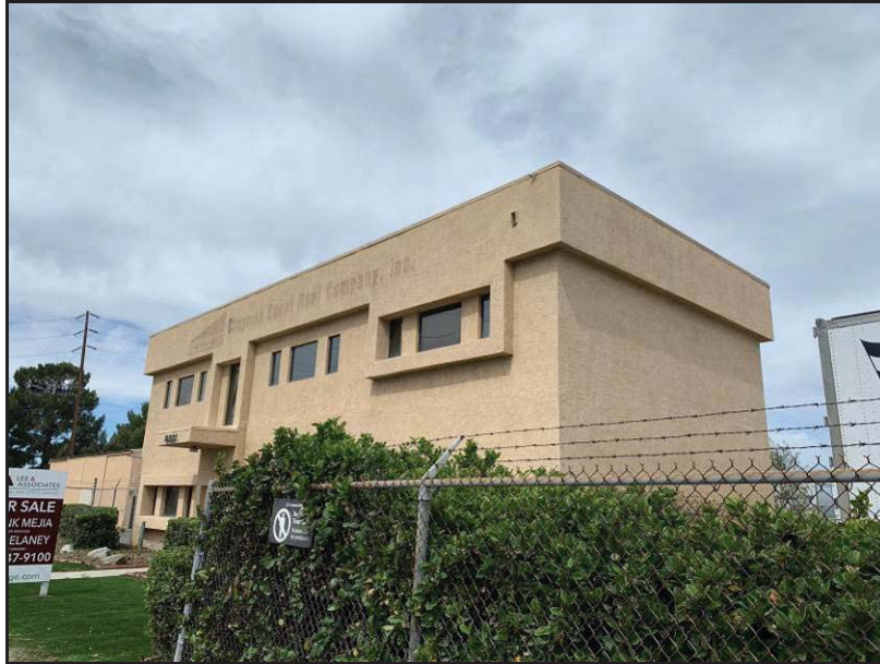
Image 3. The south and east façades of the office building, view toward the northwest.
