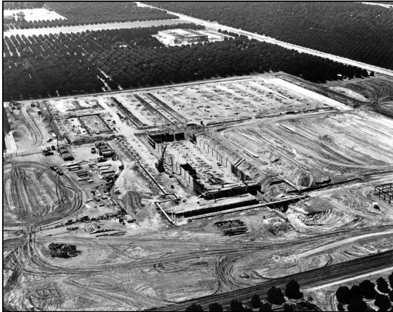
Figure 5. The Kimberly-Clark plant under construction, 1955.
