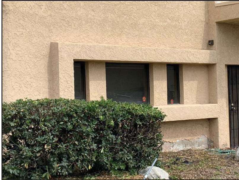
Image 5. The west façade of the office building, view toward the east.
