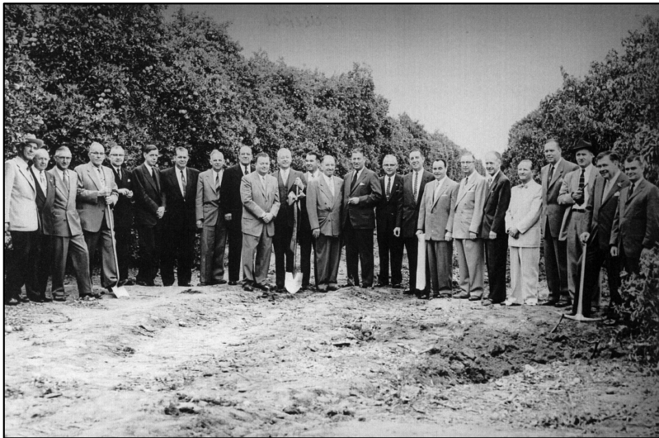
Figure 4. Groundbreaking in an orange orchard for the Kimberly-Clark Fullerton Plant, 1955. Source: Albert Launer Memorial History Room, Fullerton Public Library.
