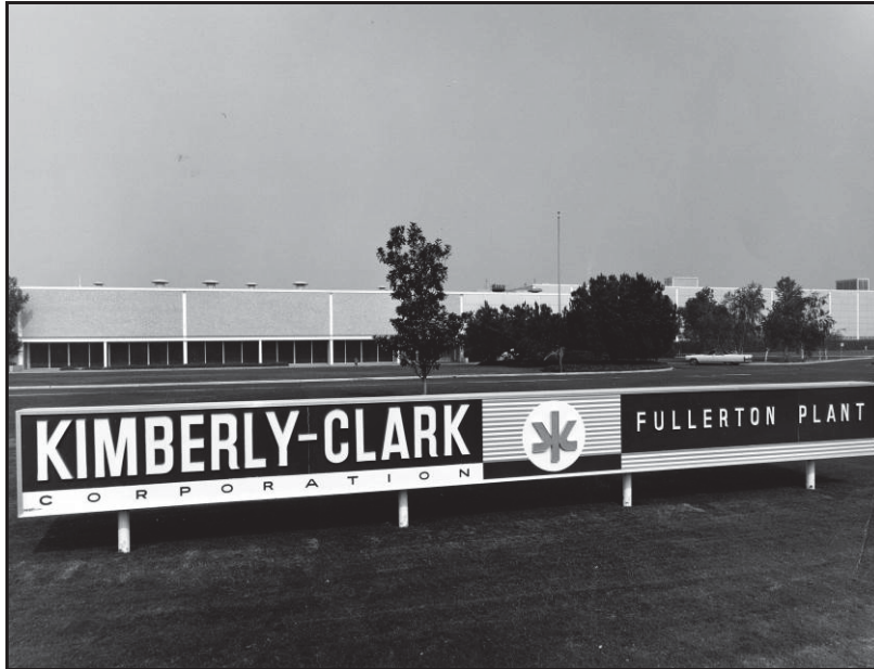
Image 3. Primary façade (south) of the Kimberly-Clark sign and plant, view toward the north, showing original building and landscape, undated. Source: Albert Launer Memorial History Room, Fullerton Public Library.
