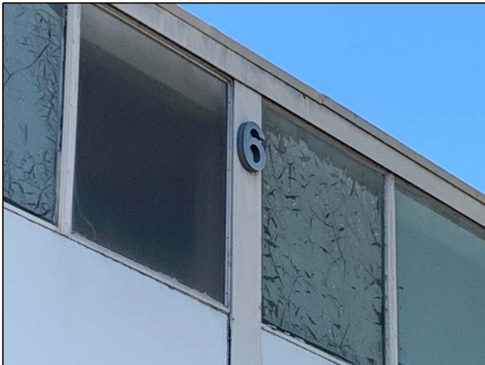
Figure 29. Detail of original windows at the north façade of the building.
