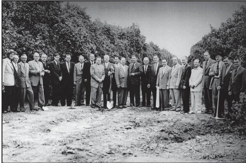
Image 1. Groundbreaking in an orange orchard for the Kimberly-Clark Fullerton Plant, 1955. Source: Albert Launer Memorial History Room, Fullerton Public Library.
