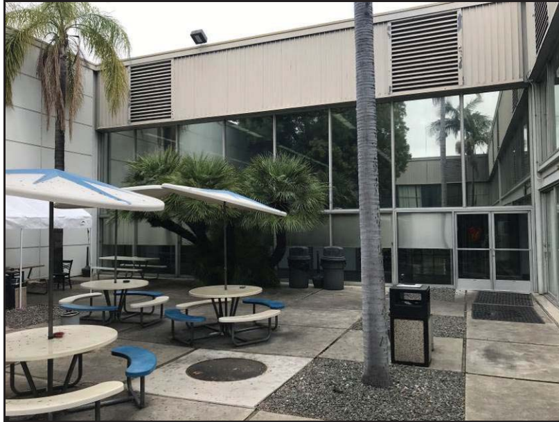
Image 23. The courtyard behind the original primary entrance, view toward the northwest.
