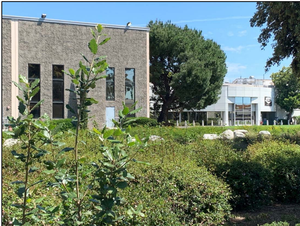
Figure 21. Detail of the south façade to the west of the primary entrance, view toward the northeast.
