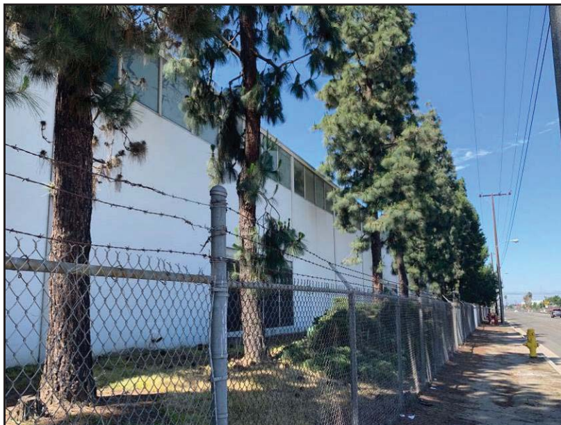
Image 16. Detail of the north façade of part of the original building along Kimberly Avenue, view toward the southwest.
