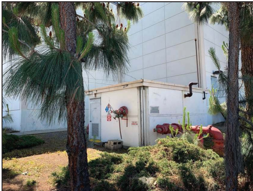
Image 18. The utilitarian shed at the southwest corner of South Acacia Avenue and Kimberly Avenue, view toward the southeast.
